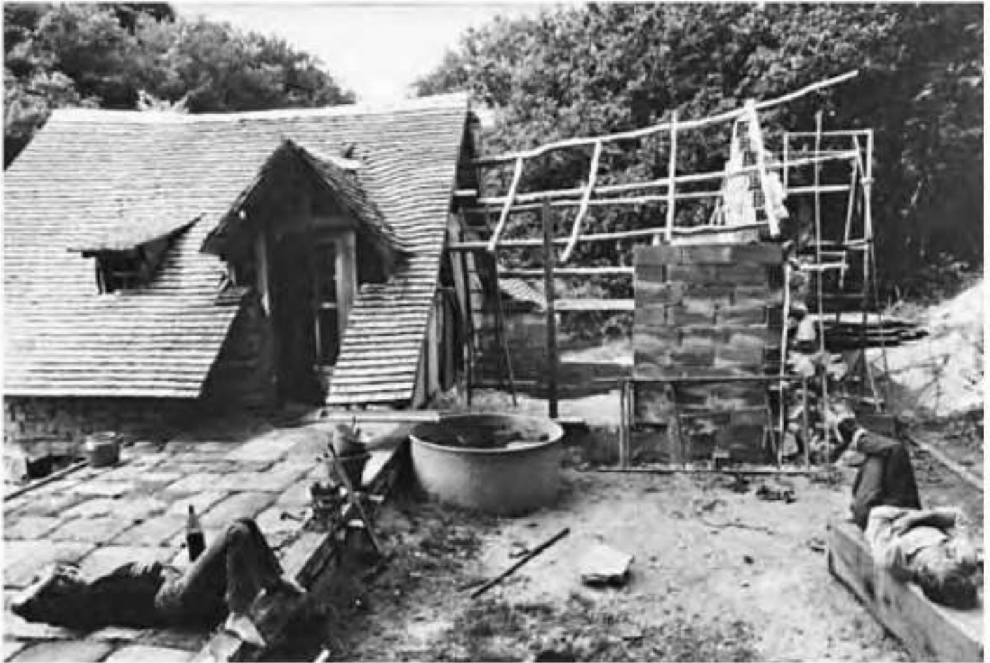
House under construction, La Vallée.
